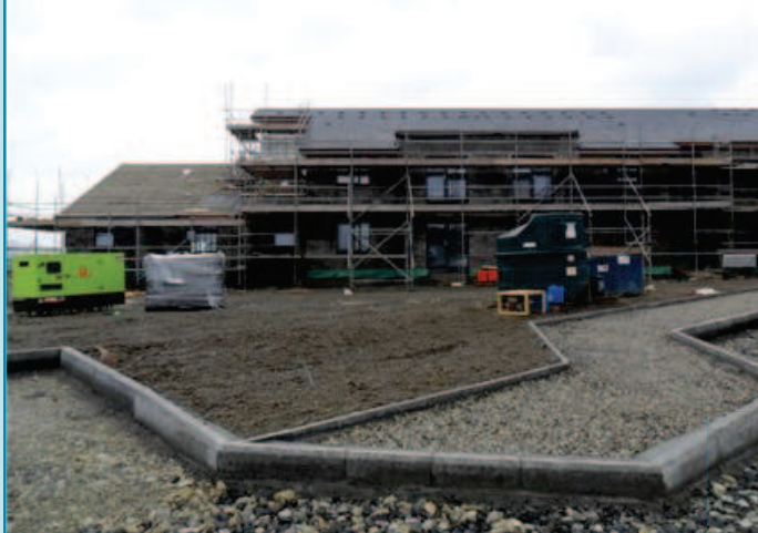
Mull Progressive Care Centre under construction
